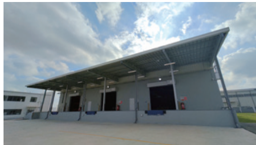
General view of the newly built warehouse
