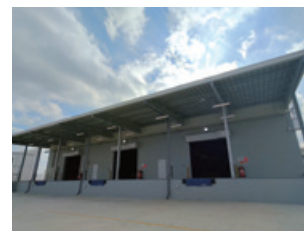
The first Japanese-quality hazardous materials warehouse in Vietnam
