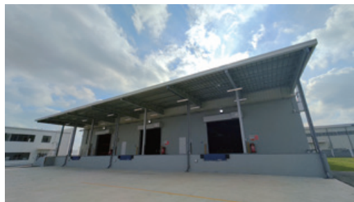
General view of the newly built warehouse
