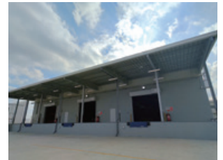
The first Japanese-quality hazardous materials warehouse in Vietnam
