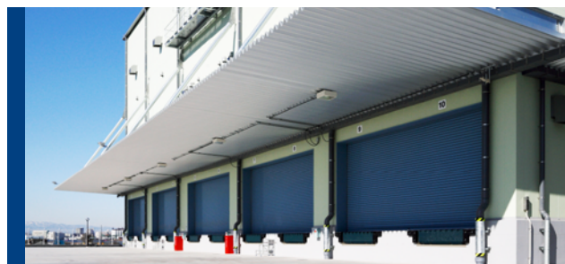
General goods warehouse (controlled / ambient temperature)
