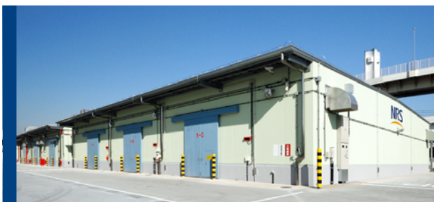
Hazardous materials warehouse (controlled/ambient temperature)
